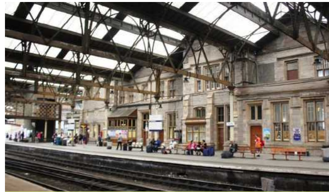
Existing Roof Structure within Station
