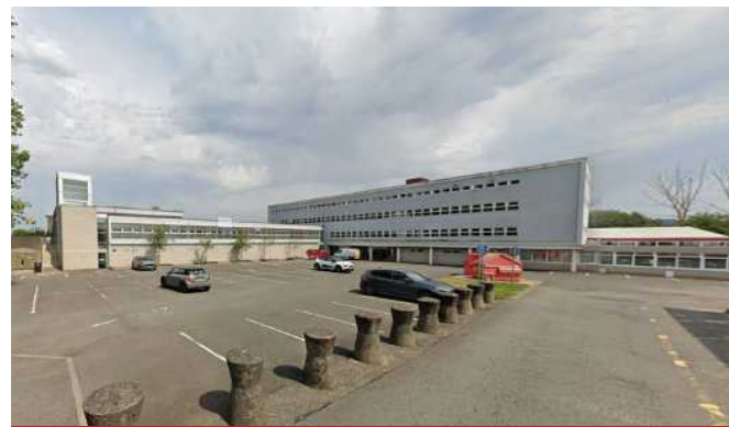
UHI Perth - Goodlyburn Building
