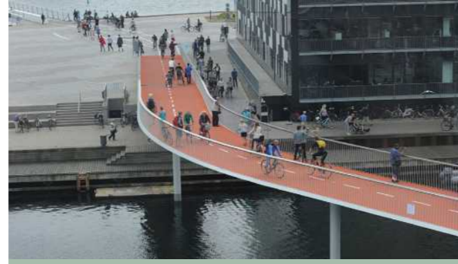
Active Travel Bridge
