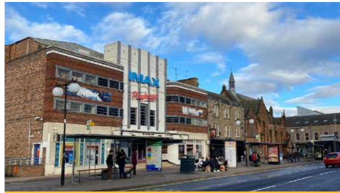
Key buildings: cinema, bar/restaurant and church
