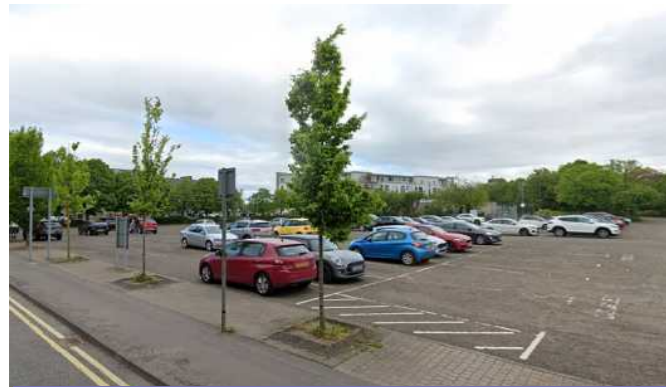
Existing Thimblelow Car-park
